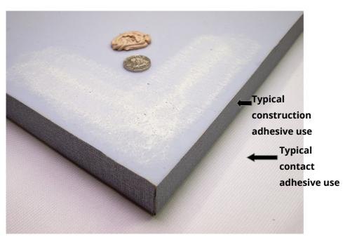
When pressing into position, use a clean wooden trowel or similar to spread the force and prevent damaging the surface. Push in the area that the construction adhesive has been applied.
